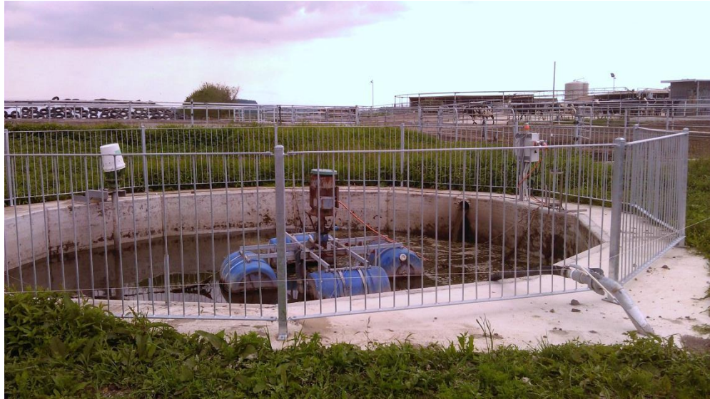
Photo One: A fully fenced sump
