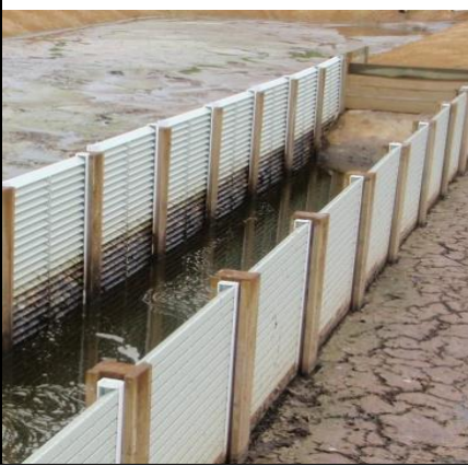
Photo Two: Screw press separator and sealed concrete receiving area.
